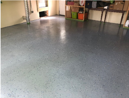
12088 Brewster garage floor after painting
