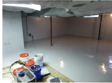
12036 Brewster basement after first application of RetroCoat
