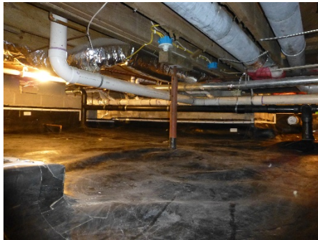
12070 Boston Post liner installed in crawl space
