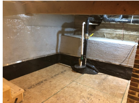
12131 Boston Post basement after RetroCoat
