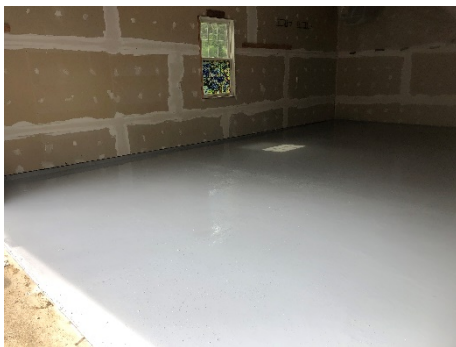
34600 Beacon Garage after RetroCoat application
