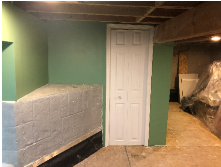
12131 Boston Post basement after RetroCoat
