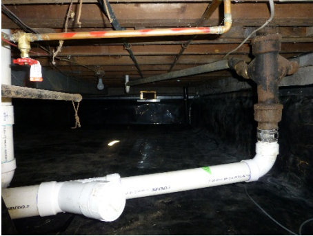
34401 Capitol new sanitary line
