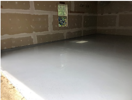
34600 Beacon Garage after RetroCoat application
