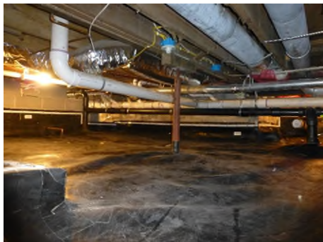
12070 Boston Post liner installed in crawl space
