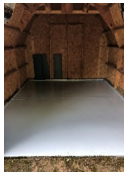
34990 Beacon RetroCoat of shed floor
