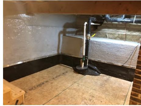
12131 Boston Post basement after RetroCoat
