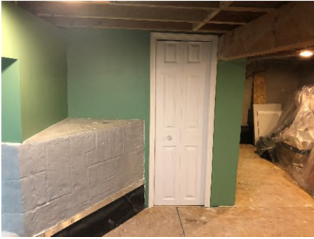
12131 Boston Post basement after RetroCoat
