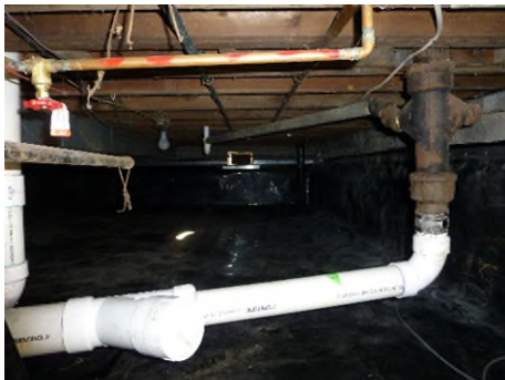
34401 Capitol new sanitary line
