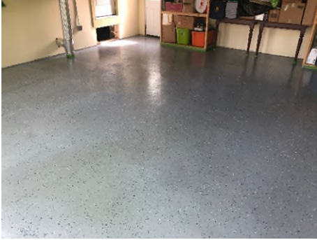
12088 Brewster garage floor after painting
