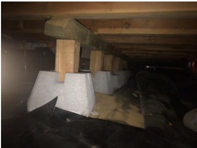
34367 Capitol structural repair
