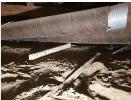
12124 Boston Post ducts need to be moved
