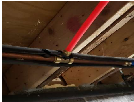
34424 Capitol New plumbing repair
