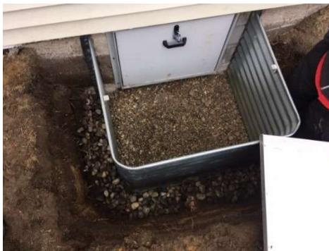
34424 Capitol new crawlspace access door
