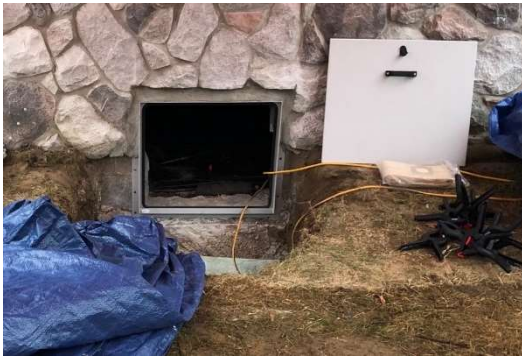
34644 Beacon new crawlspace access
