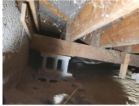
12124 Boston Post structural support, inaccessible space
