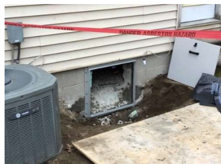
12124 Boston Post new crawlspace access
