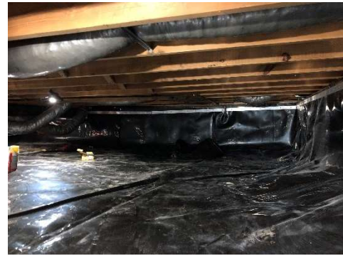
34644 Beacon barrier installation
