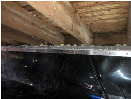
34424 Capitol sealed crawlspace
