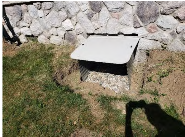
Modified crawlspace entrance on June 17, 2020.
