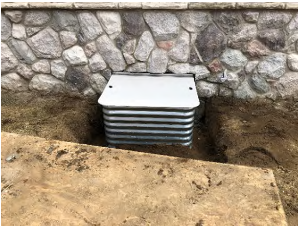
Constructed entrance on March 16, 2020.
