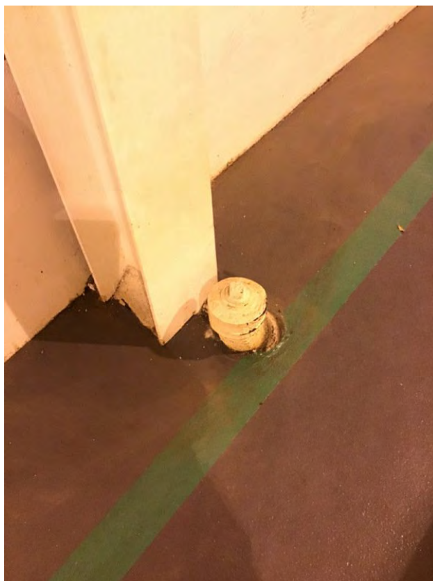
Clean out on west wall near R56
