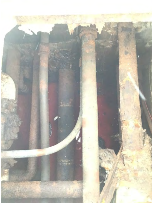
Vault 2, open pipe coming in from the west
