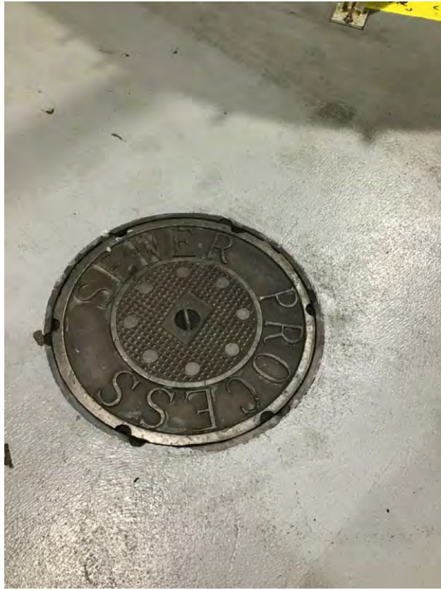
Manhole 26, near B78
