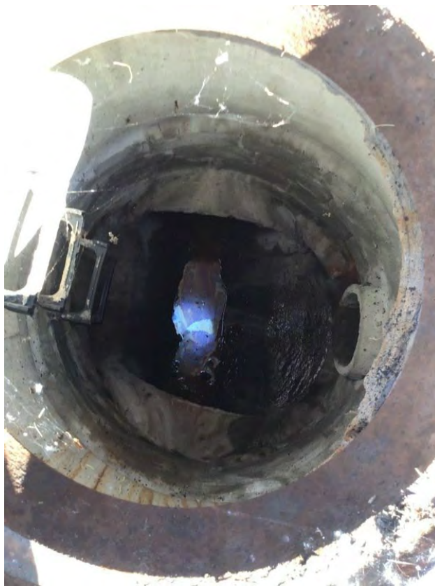
Sheen on top of stagnant water in STMH 1066
