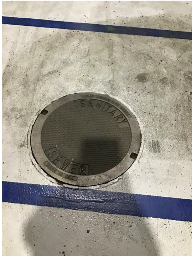
Manhole 19, near J92
