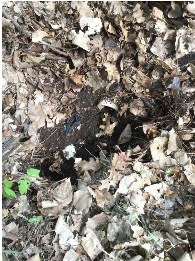
STMH 1219 inlet piping to N 12"
