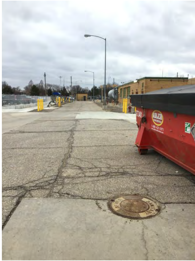
Manholes 3A and 3B, photo looking south
