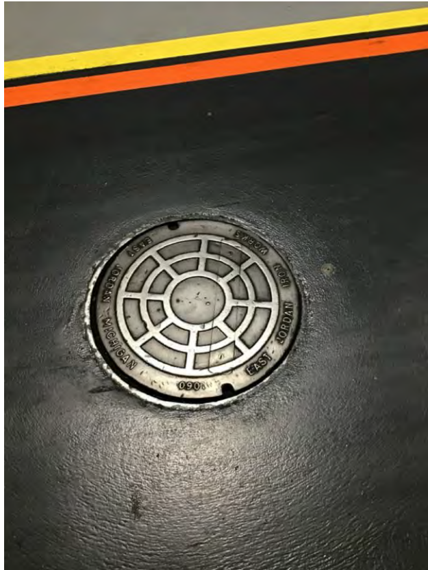
Manhole 21, in traffic way near H100
