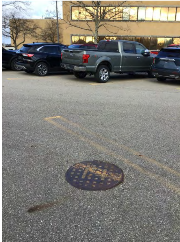
Southwest corner of office/plant, unable to open manhole
