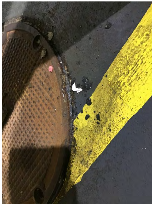
East wall manhole
