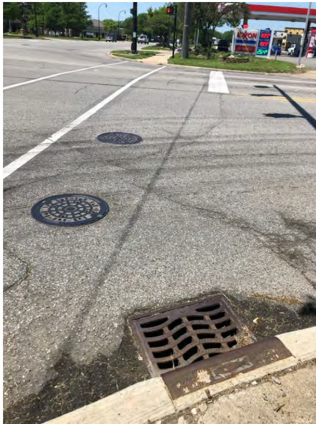
Catch basin in Plymouth and Levan intersection. Runs west into storm manholes
