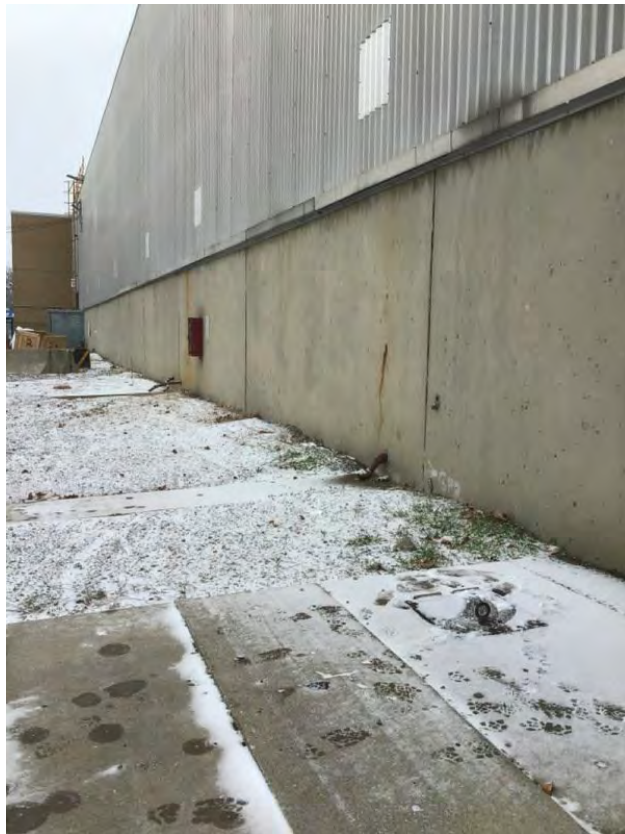
Vault 1 at southeast entrance to plant
