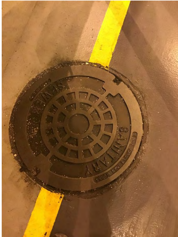
Manhole 2, east side of plant
