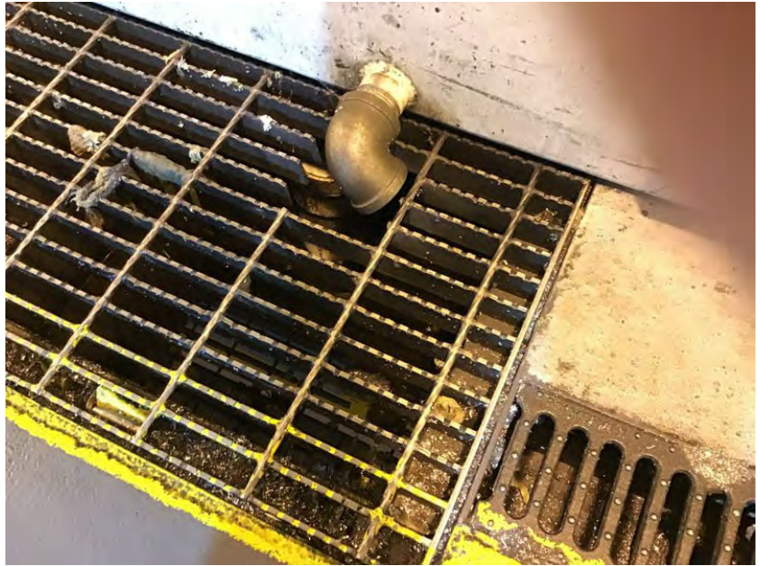
Floor drain at F42
