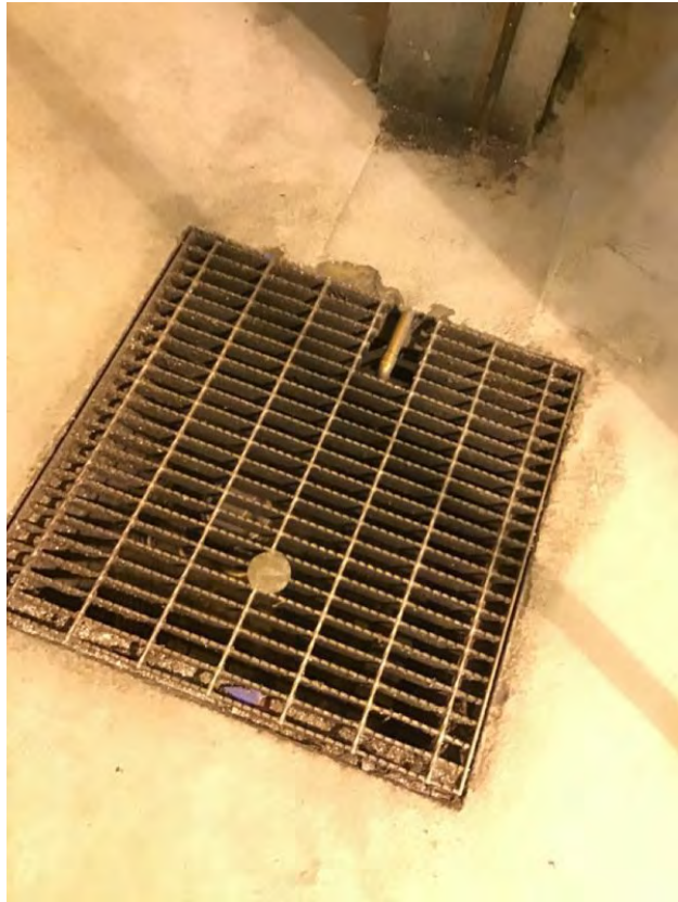
Floor drain with a clean out at F46
