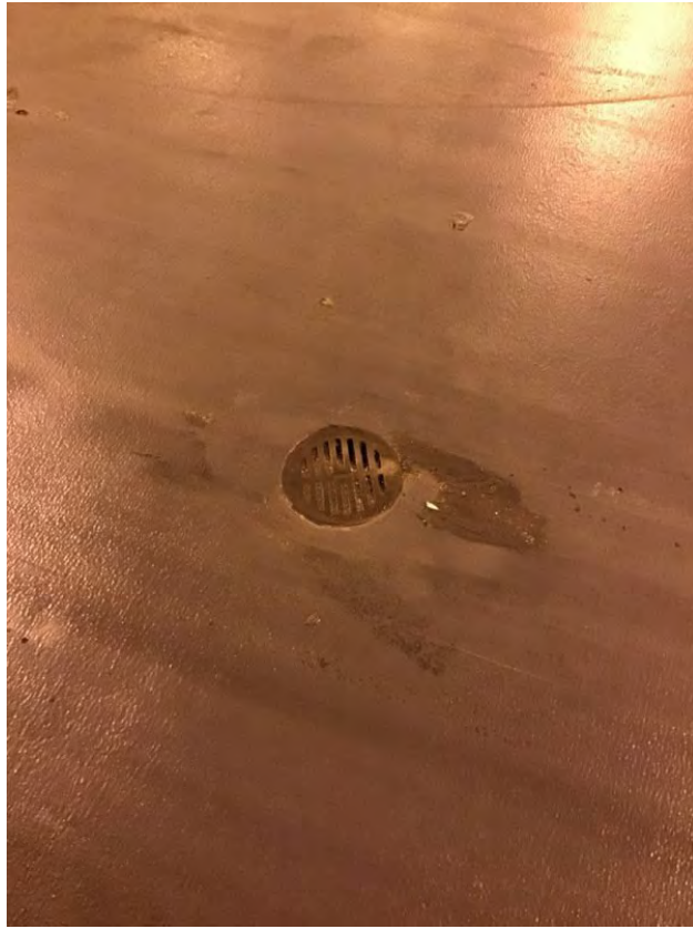
Filled floor drain near R64
