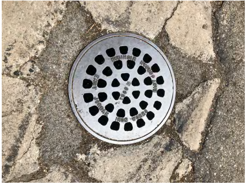
Catch basin in Levan Wine Shoppe parking lot. Pipes running north and south. Catch basin of this one runs only south
