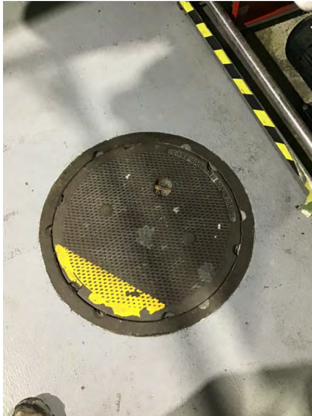
Manhole 12 near H6
