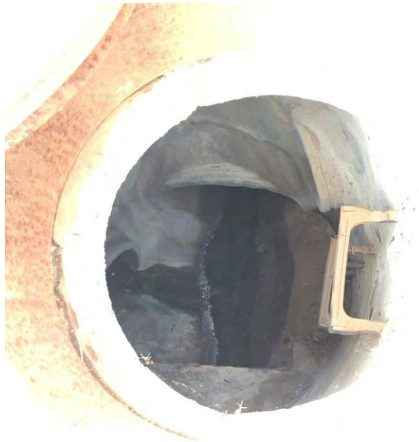
MH-1088 concrete bottom
