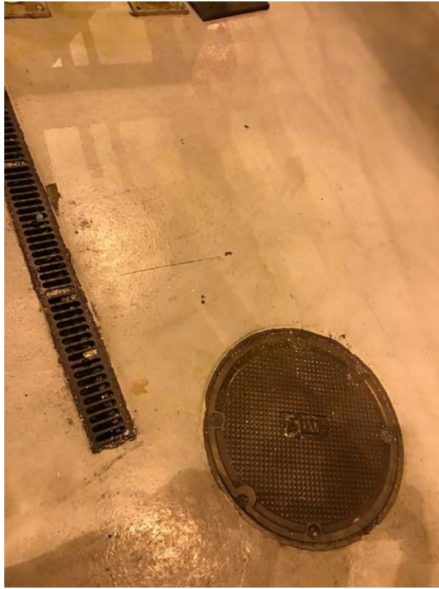
Manhole 4, with floor drain next to it
