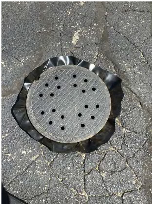
Vapor barrier on STMH 1066
