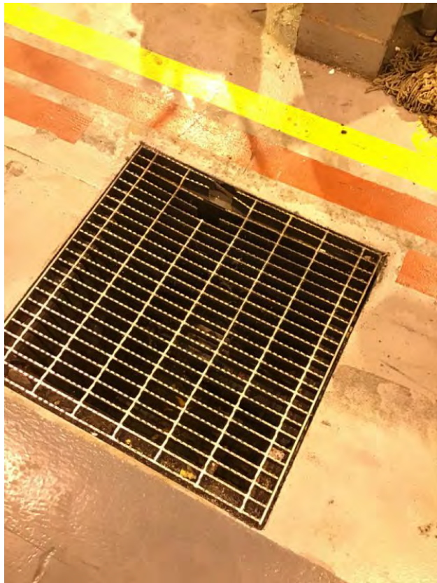
Floor drain at B46
