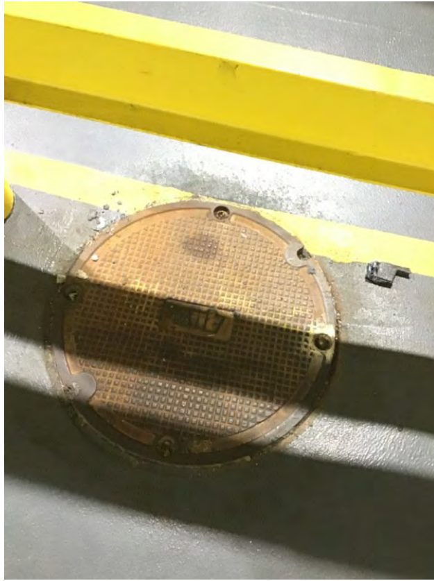
East wall manhole
