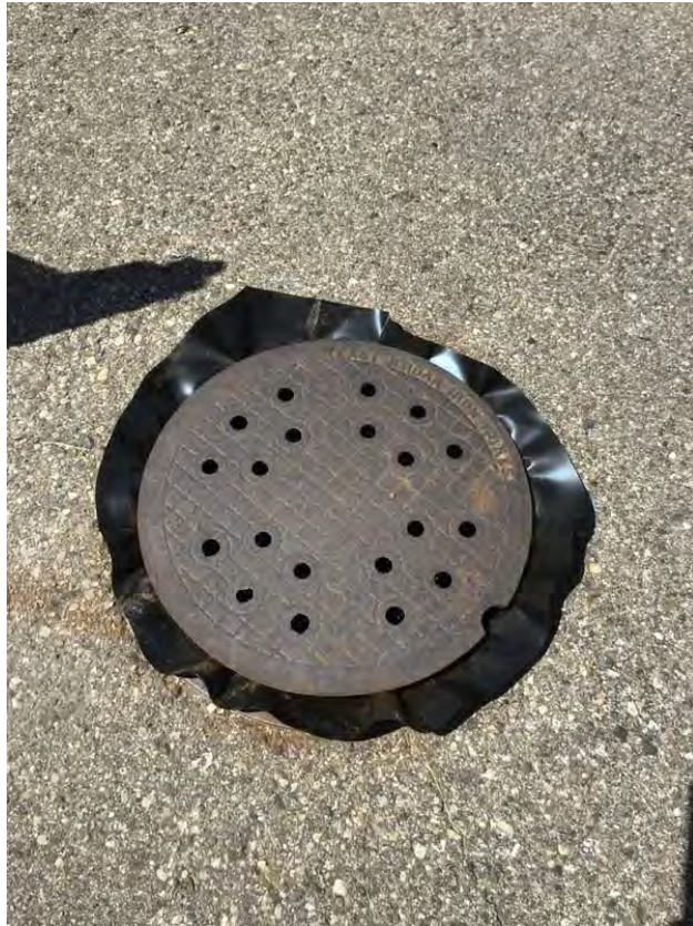
Vapor barrier on STMH 1041
