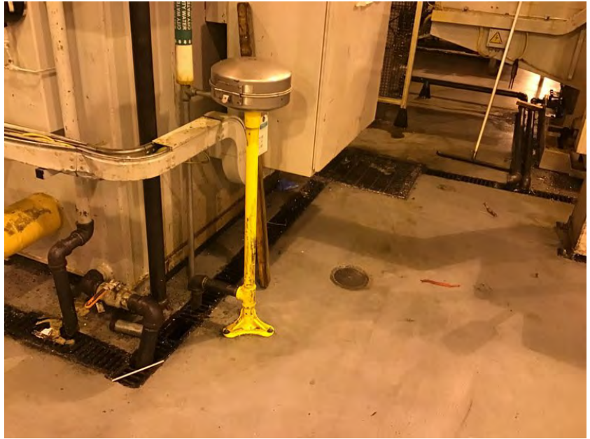
Floor drains around machines
