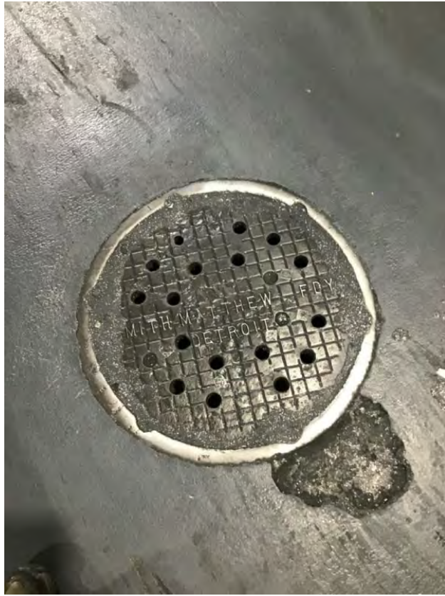
Manhole 24, in traffic way near H82
