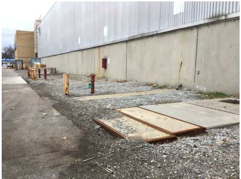
West of cylinder tanks 10-14, no manholes, photo looking south
