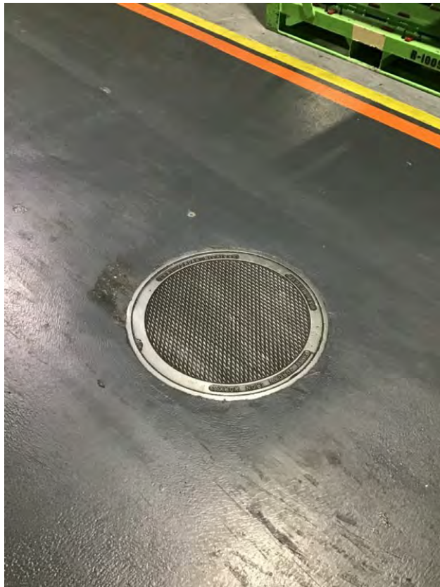
Manhole 17, located in traffic way near S88
