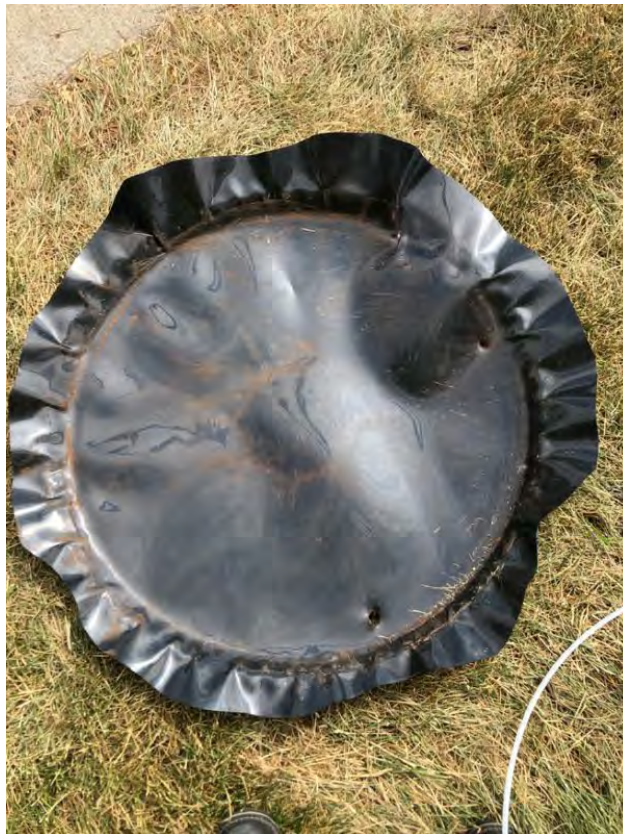
Vapor barrier at SL-2 still intact (2 holes are from us poking holes to sample)
