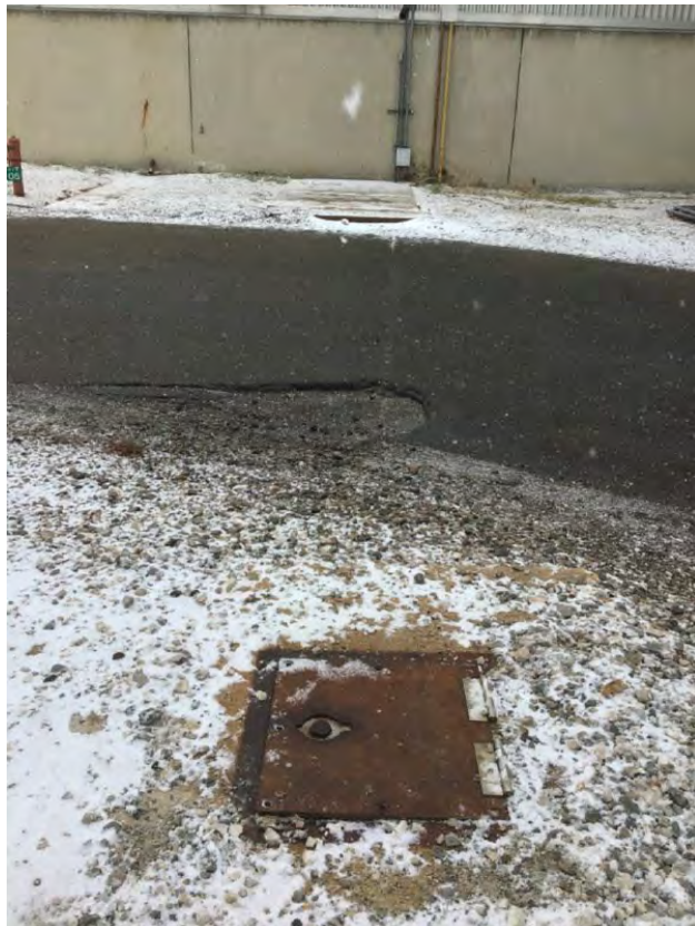
Vault 2, southeast plant entrance
