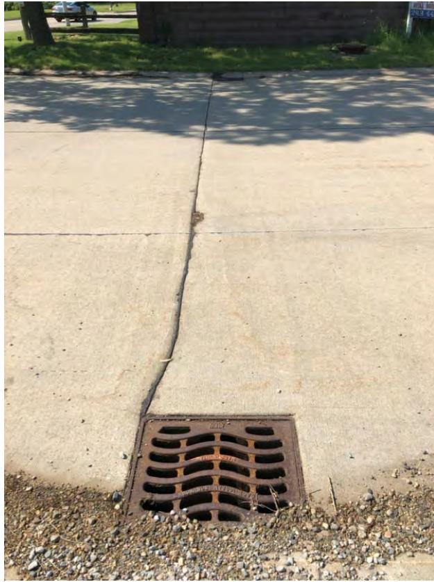
North storm drain on Rosati
