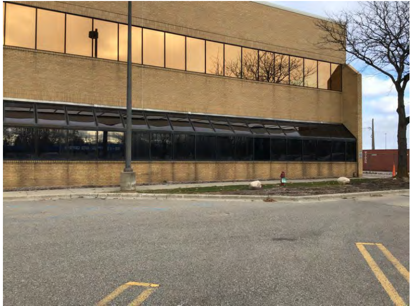
Southeast corner of office/plant
