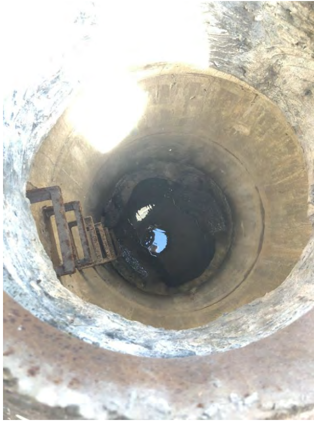
Storm man hole north of Plymouth along Levan
