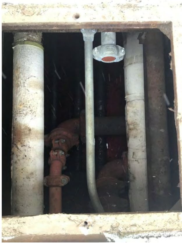
Inside of vVault 1 at southeast plant entrance
