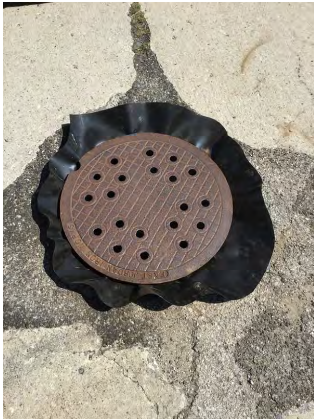
Vapor barrier on STMH 1088
