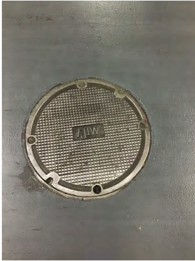
Manhole 20, in traffic way near H104
