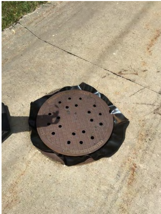
Vapor barrier on STMH 1171
