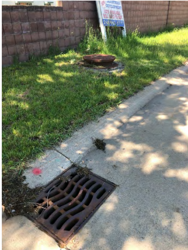
South storm drain on Rosati
