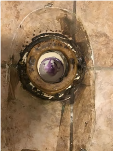
Existing wax ring and caulk seal around removed toilet
