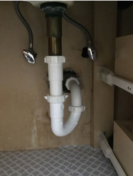
Inspected P-trap under the bathroom sink
