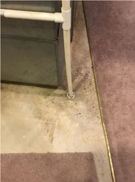
Inspected P-trap at the furnace condensate drain below the concrete floor
