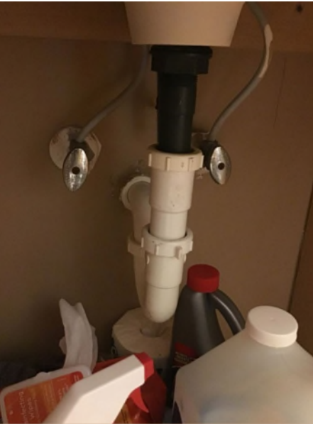
Inspected P-trap under the restroom sink
