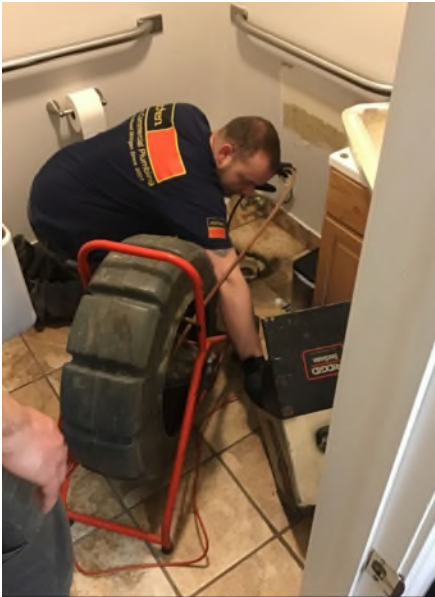
Sewer lateral inspected via camera from the restroom toilet
