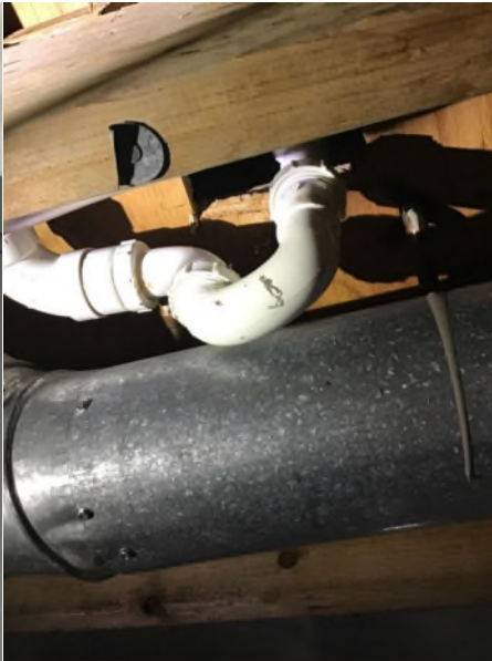
Inspected P-trap under the shower in the basement
