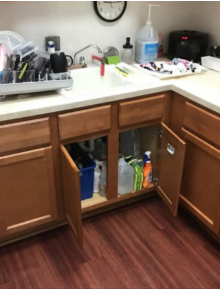
Inspected P-trap at the kitchen sink
