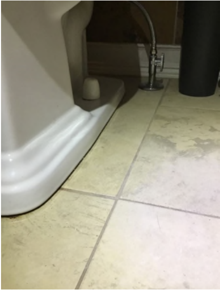
Existing toilet without caulk sealing around the base
