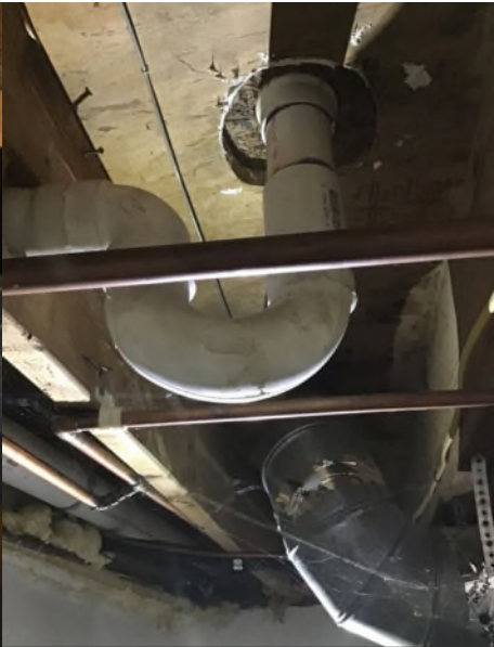
Inspected P-trap under the bathtub in the basement
