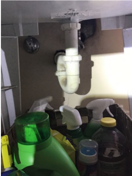
P-trap inspected under the laundry room sink
