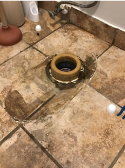
New wax ring installed on toilet flange
