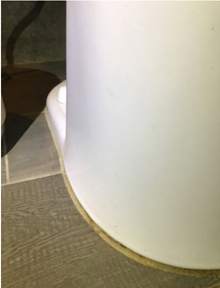
Toilet grouted to the tile floor
