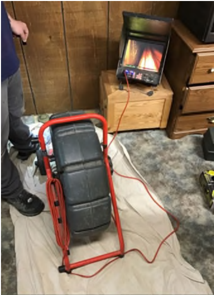
Interior cleanout inspected lateral with a camera
