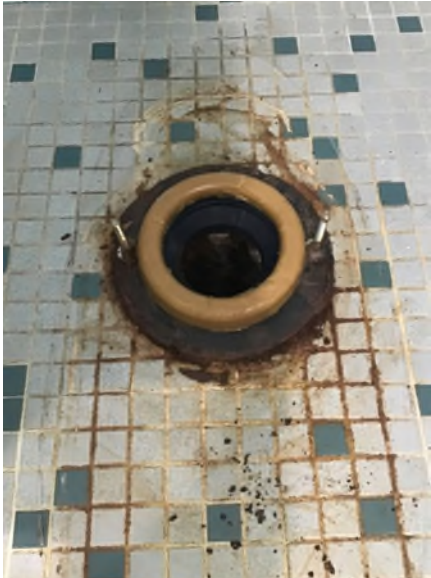
New wax ring installed on toilet flange
