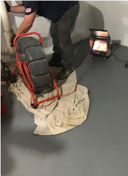
Interior cleanout inspected lateral with a camera
