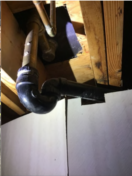
Inspected P-trap under the bathtub in the basement
