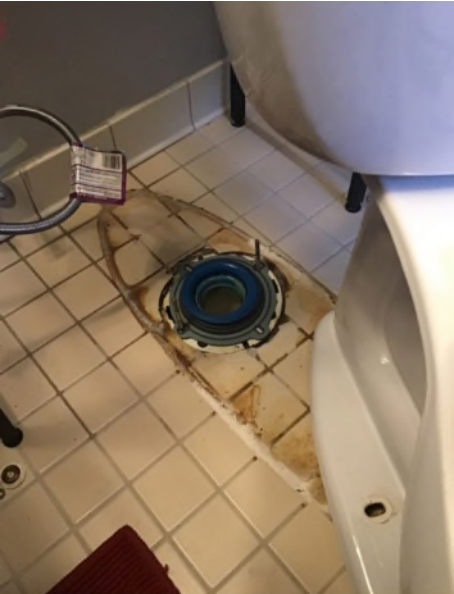
Inspected wax-less toilet gasket under toilet
