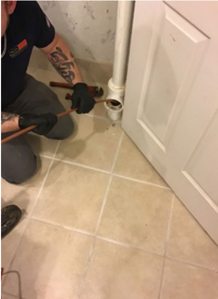
Interior cleanout inspected lateral with a camera
