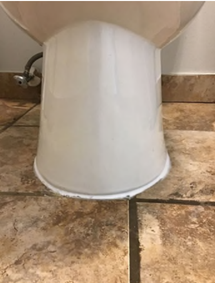
Toilet reinstalled and new caulk applied around the base
