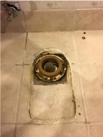
New wax ring installed on toilet flange
