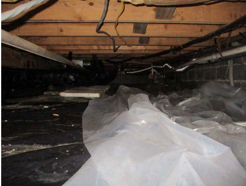
Exhibit 2. Crawlspace at 34880 Capitol Street.
