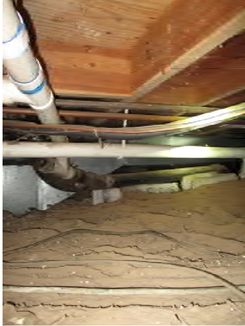
Exhibit 2. Crawlspace at 34367 Capitol Street.
