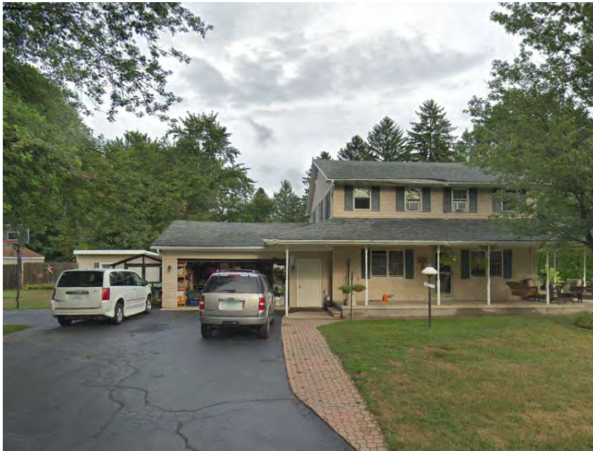
Exhibit 1. Front view of the residence at 12017 Brewster Street
