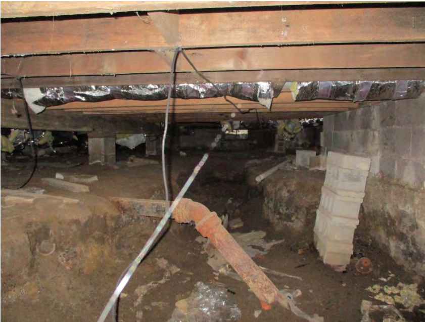
Exhibit 2. Crawlspace at 34591 Beacon Street
