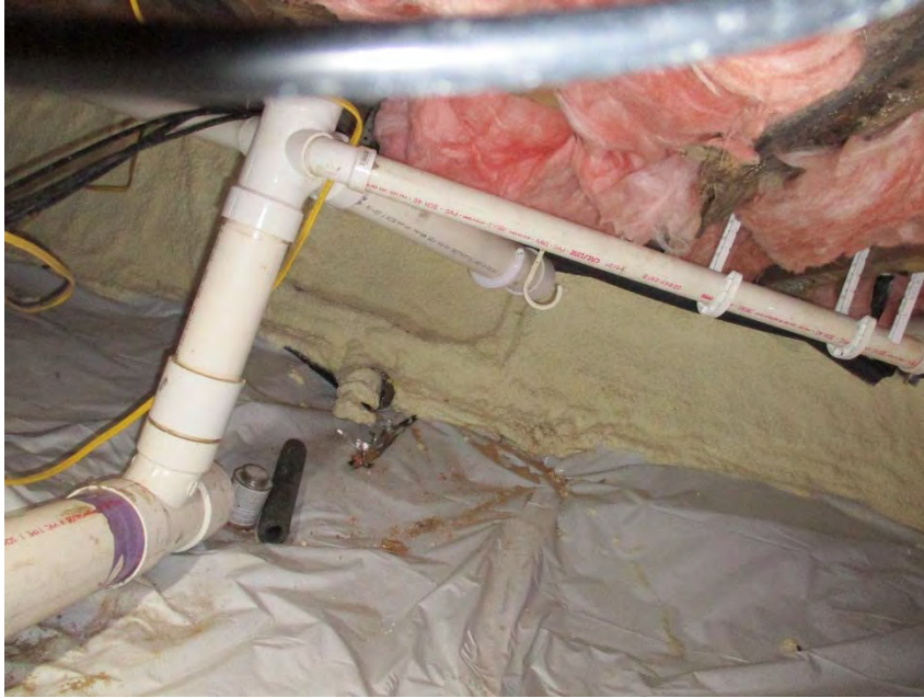
Exhibit 2. Crawlspace at 34682 Beacon Street
