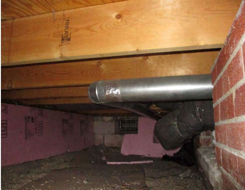
Exhibit 2. Crawlspace at 34990 Beacon Street
