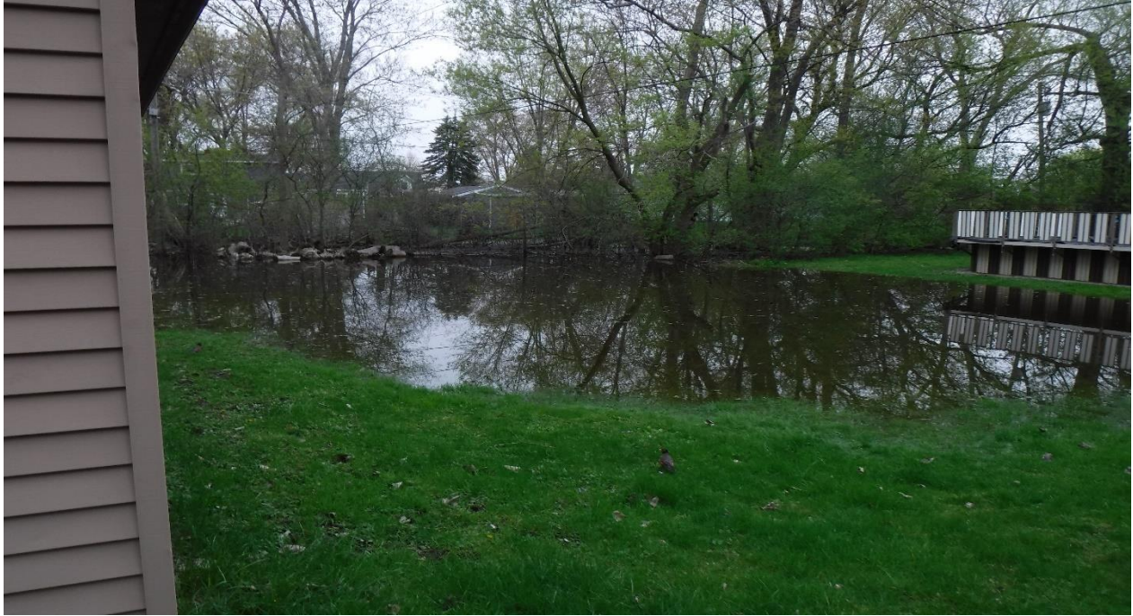
Photo 3 - Flooding Conditions Near 34450 Beacon
