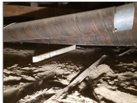
Numerous heating ducts lying on the floor or hanging with less than 10” of clearance below.
