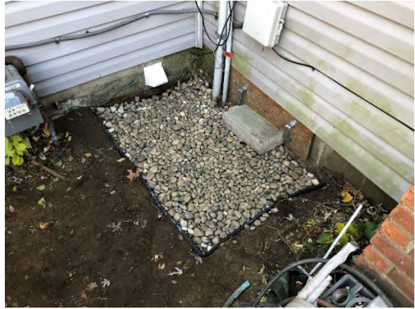
Crawlspace entrance modified to prevent water from entering.
