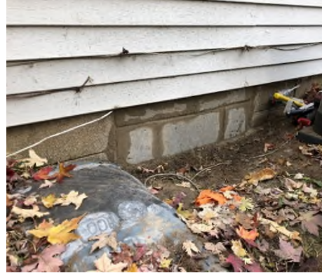
Photo of the window after it was sealed.
