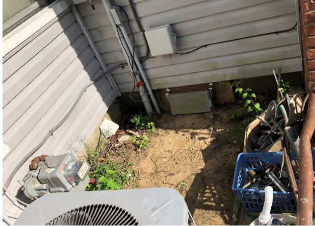
Previous crawlspace entrance.
