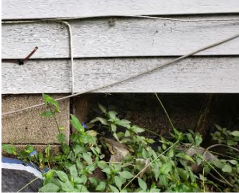
Photo of the crawlspace window before.
