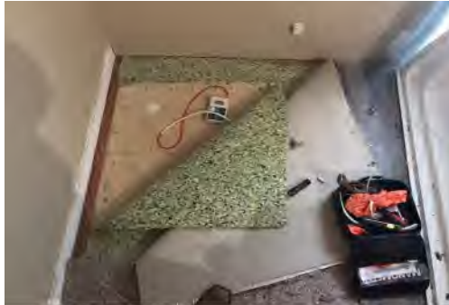
elevated subfloor, west living space.
