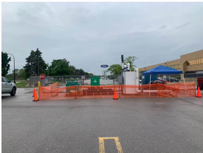
Exhibit 1 - Sanitary Sewer Vapor Extraction System
