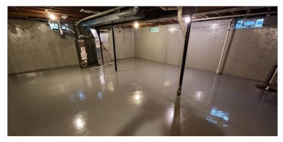
The third annual OM&M event was completed on May 17, 2023 after repairs to the Retro-Coat<sup>™</sup> were completed. All monitoring points achieved the performance metric established by EGLE of -0.02 iwc.
