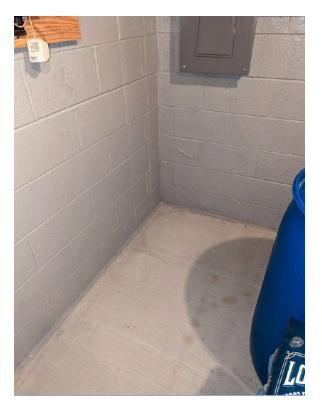
A system inspection was completed on June 7, 2023 following the caulking repair and all monitoring points achieved the performance metric established by EGLE of -0.02 iwc.
