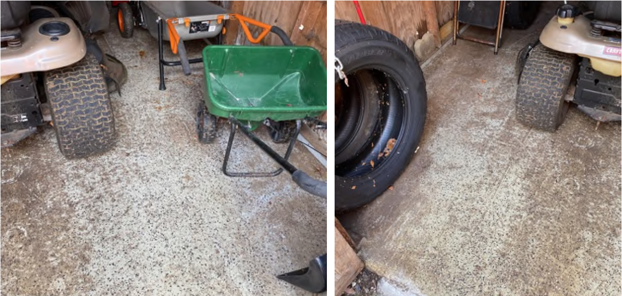
12075 Brewster - Detached shed with Retro-Coat®, photograph taken on April 17, 2024.
