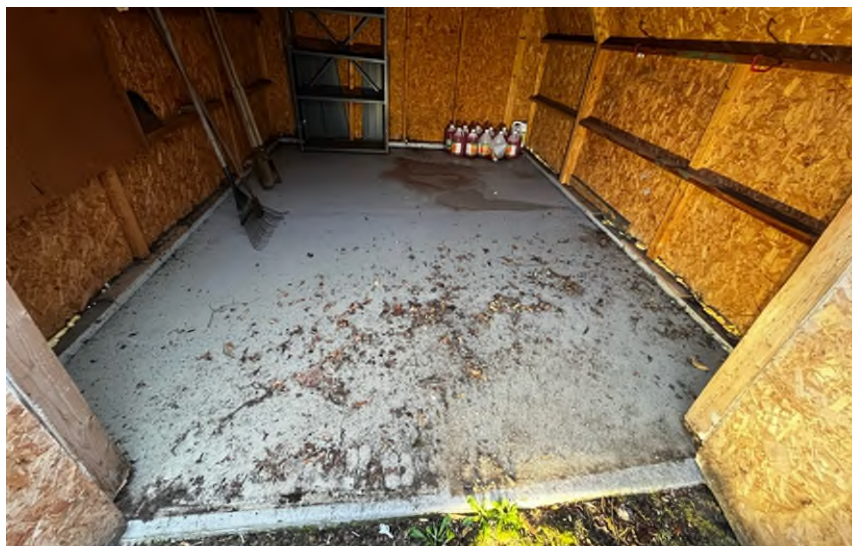
34990 Beacon detached shed with Retro-Coat®, photograph taken on March 14, 2024.
