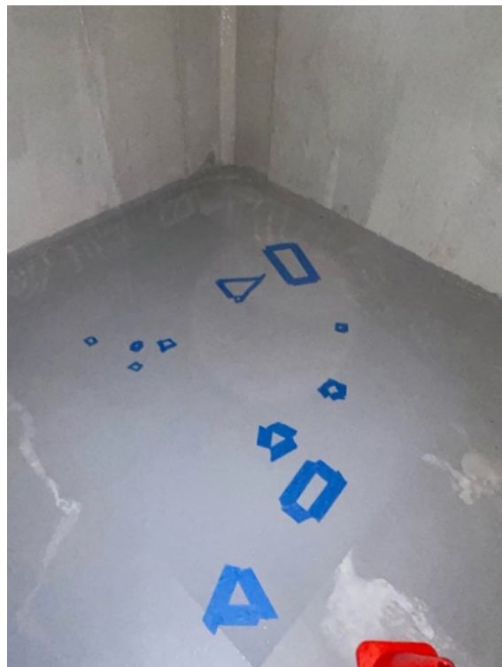
34940 Beacon – Two photographs showing the cured Retro-Coat® and the pinhole depressions in the recently applied Retro-Coat®. Photographs taken on April 25, 2024.
