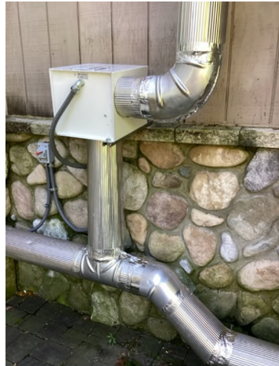
12131 Boston Post: Removal of the damaged fan (left). Replacement AMG Force Fan installed (right).
