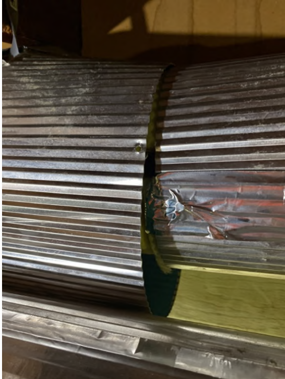
34550 Beacon: Damaged insulation and jacketing (left). Repaired insulation and jacketing (right).
