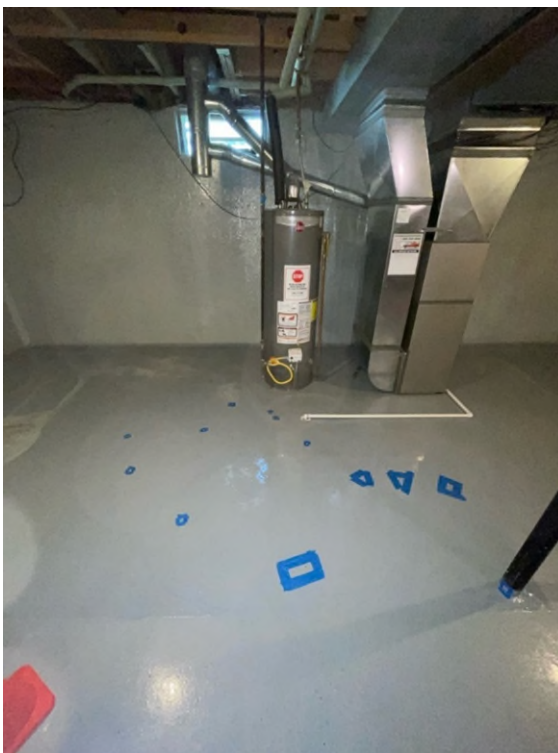
34940 Beacon – Two photographs showing the cured Retro-Coat® and the pinhole depressions in the recently applied Retro-Coat®. Photographs taken on April 25, 2024.
