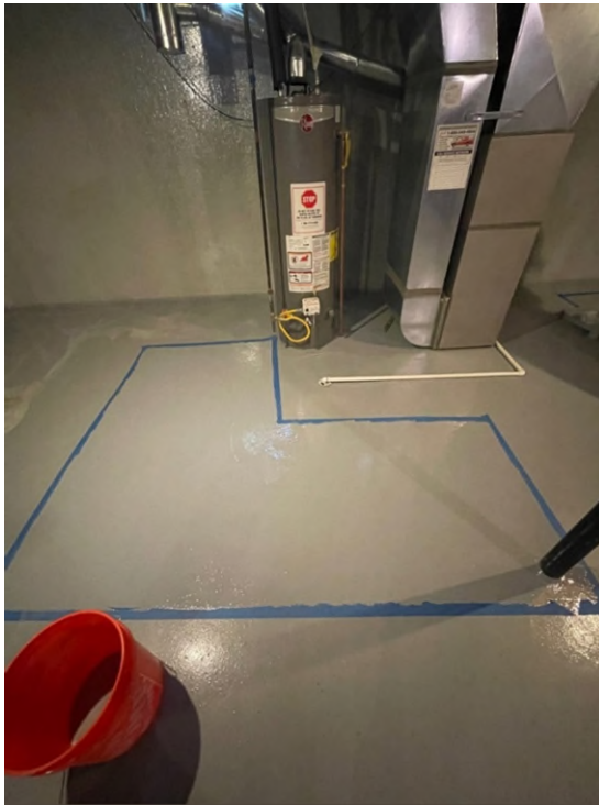
34940 Beacon – Two photographs showing the applied Retro-Coat® in the western portion of the basement. Photographs taken on April 24, 2024.
