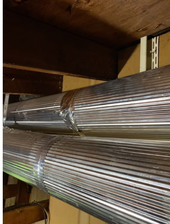
34550 Beacon: Damaged insulation and jacketing (left). Repaired insulation and jacketing (right).
