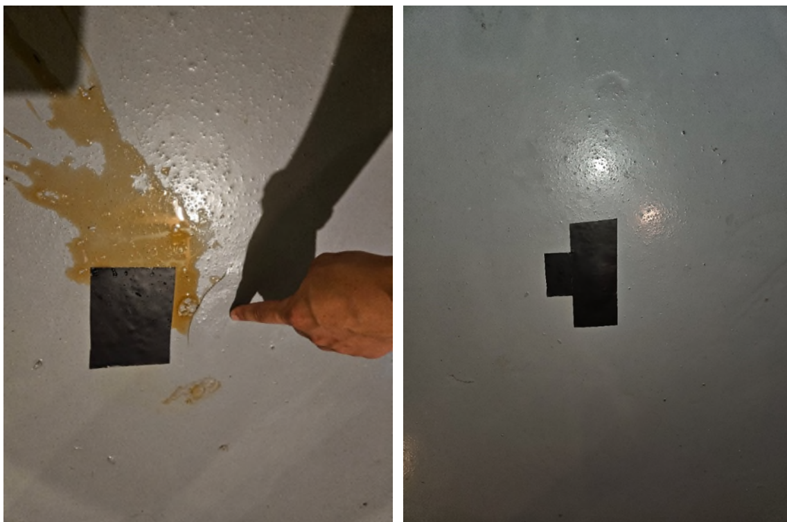
34940 Beacon – Two photographs showing the rust-colored sediment deposits (left) and completed sealing (right). Photographs taken on July 25, 2024.
