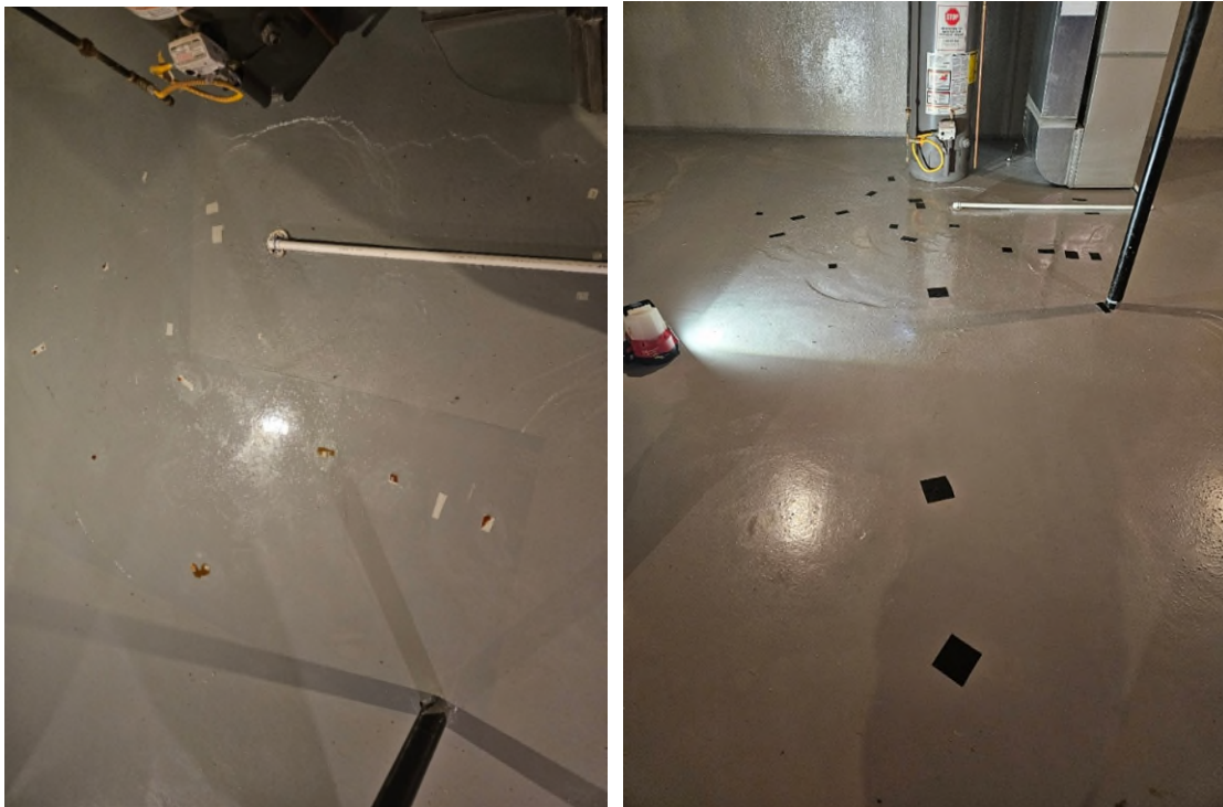
34940 Beacon – Two photographs showing the rust-colored sediment deposits (left) and completed sealing (right). Photographs taken on July 25, 2024.
