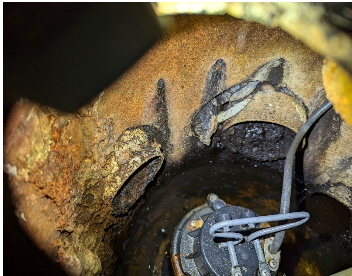
Photograph 2 – The sump basin with clogged inlet pipes.
