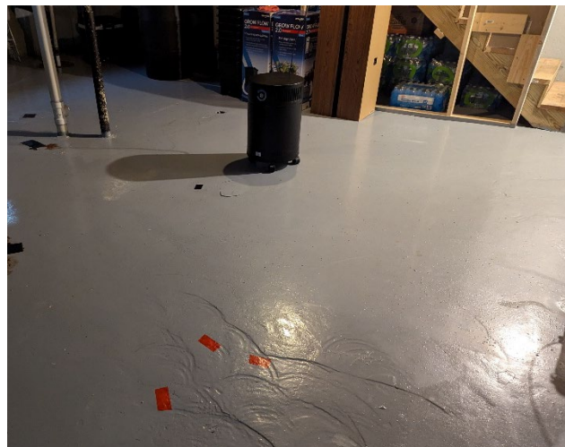
Photograph 1 – Air purifying unit deployed in the basement. Three Pinholes are sealed with plastic sheeting and red tape.
