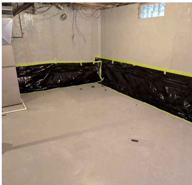
Photo 3 (left): Installation of plastic sealing the opening in the concrete floor until the replacement concrete was poured.
