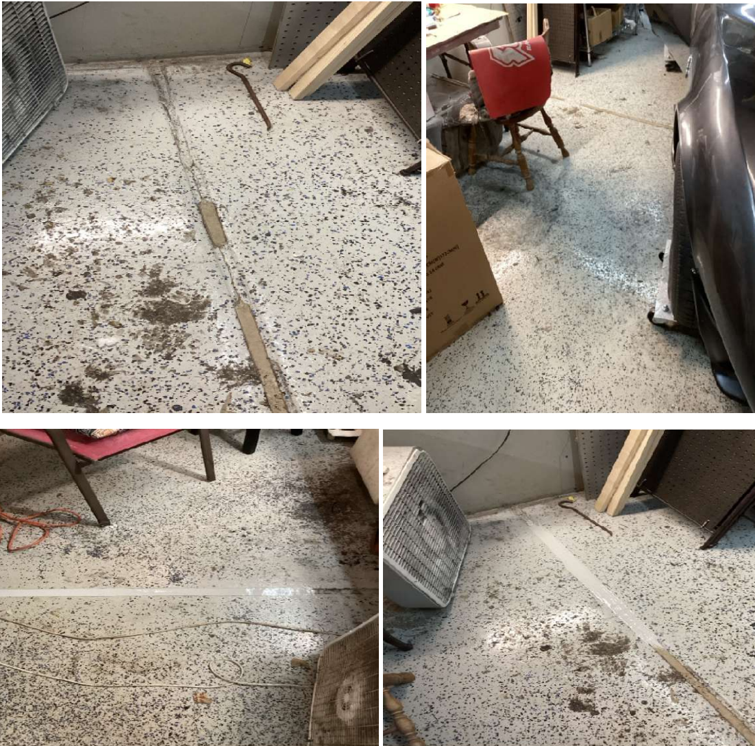
Exhibit 5: Four photographs show the small cracks and repairs to the garage Retro-coat ®.
