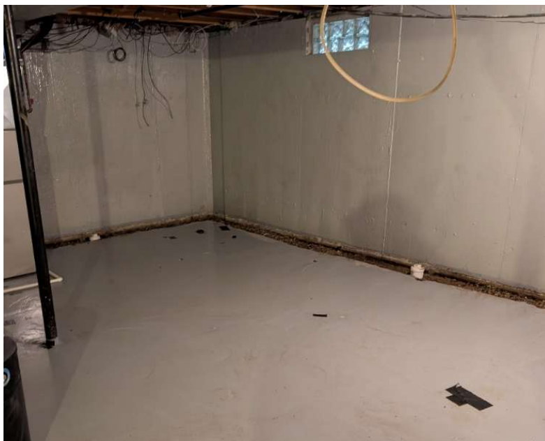
Photo 2 (right): Installation of the replacement perimeter drainage system in the basement.
