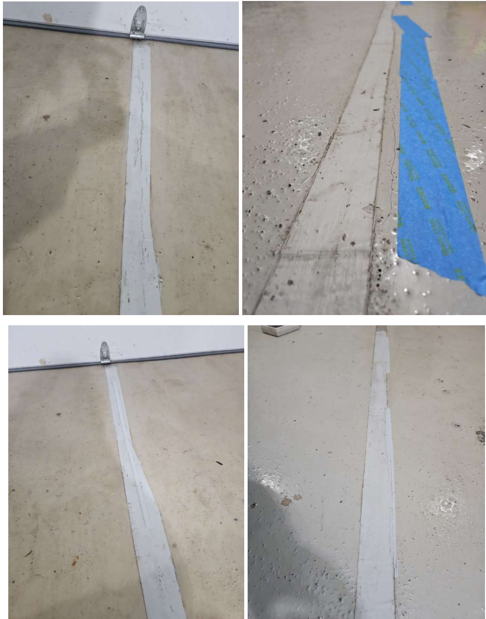
Exhibit 2: Crack repairs to the garage Retro-coat ®.
