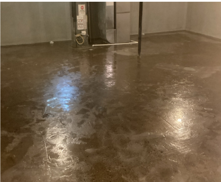
Photo 2 (right): Application of Primer MV on the basement floor.
