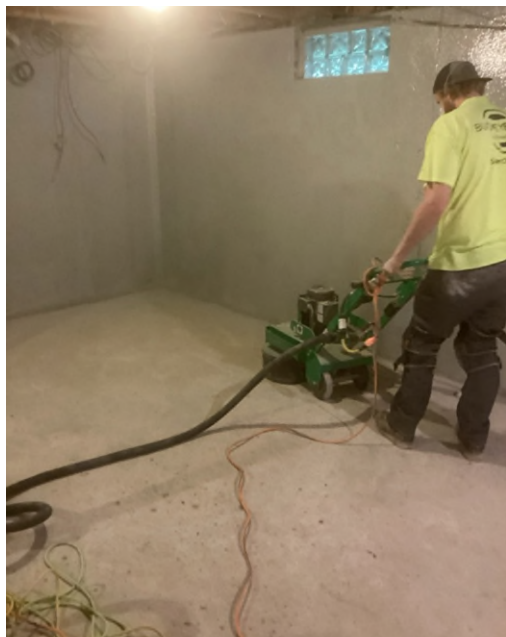
Photo 1 (left): Retro-Coat® removal using an electric grinder and HEPA vacuum attachment
