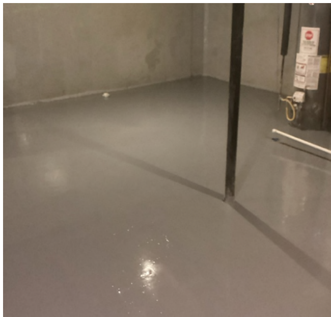
Photo 3 (left): Application of the Retro-Coat® on the basement floor.
