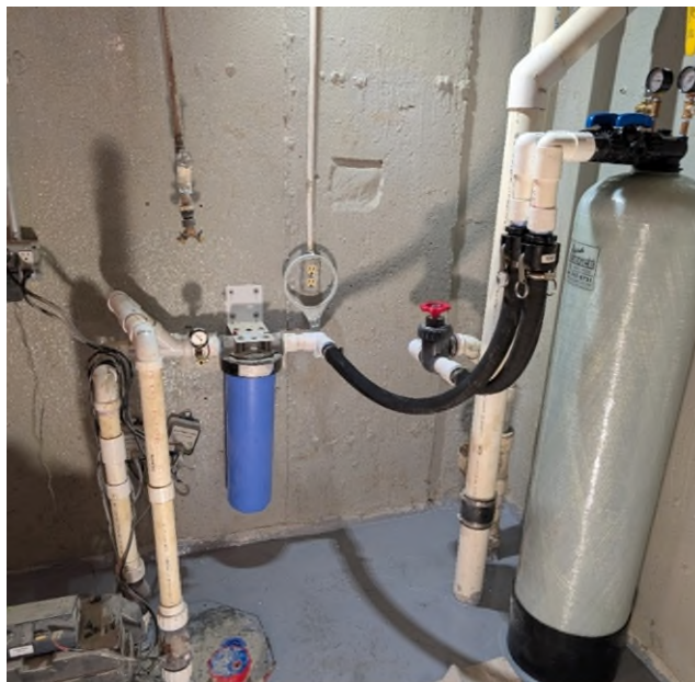
Photo 4 (right): Completed installation of the in-line sediment filter and carbon filtration tank on the sump basin discharge line.
